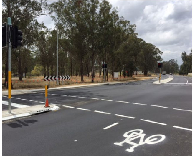
The Northern Road/Andromeda Drive, Cranebrook
