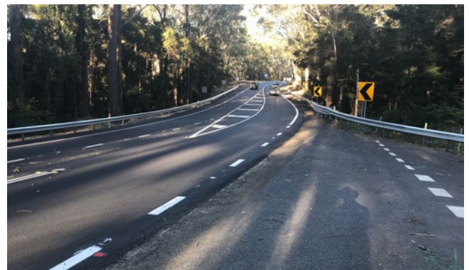
Andrews Road/Princes Highway, Basin View
