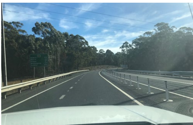
Princes Highway (between Bendalong Road & Luncheon Creek Drive), Bendalong
